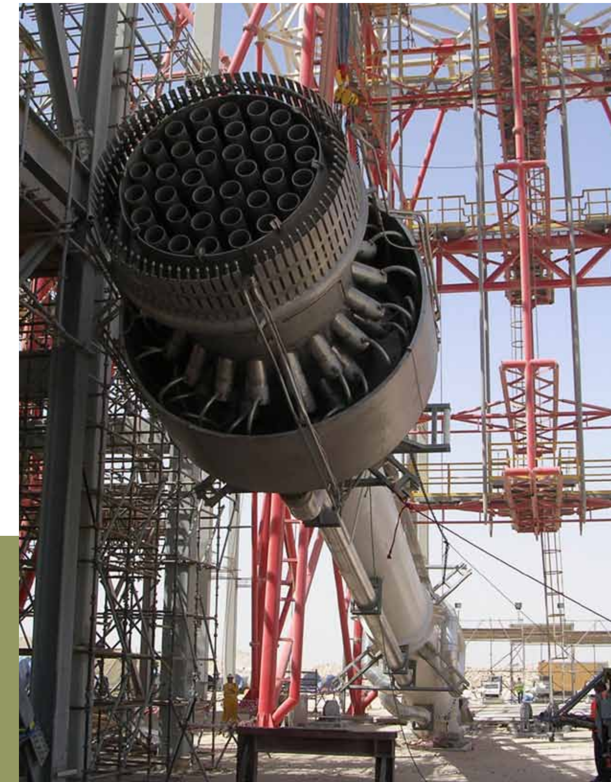
GCT-AJ-84/66C Advanced Smokeless Flare Tip being installed Qatar LNG
