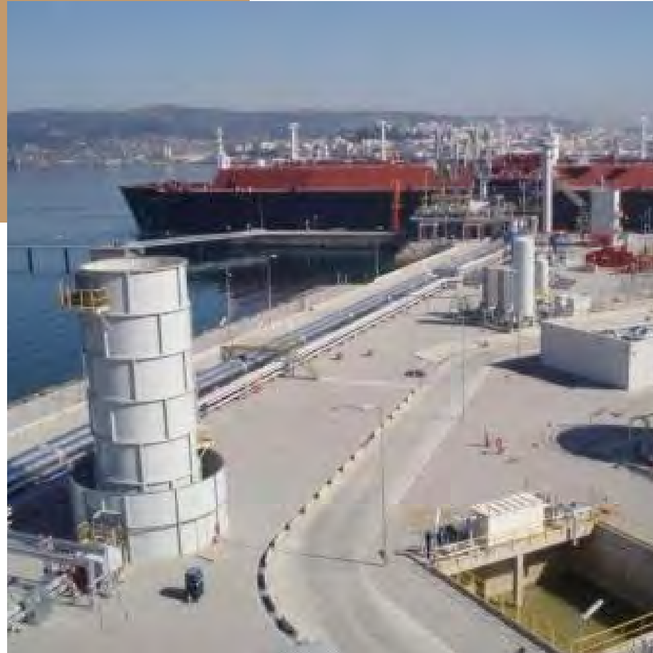
15t/h Enclosed Ground Flare Mugardos, Spain
