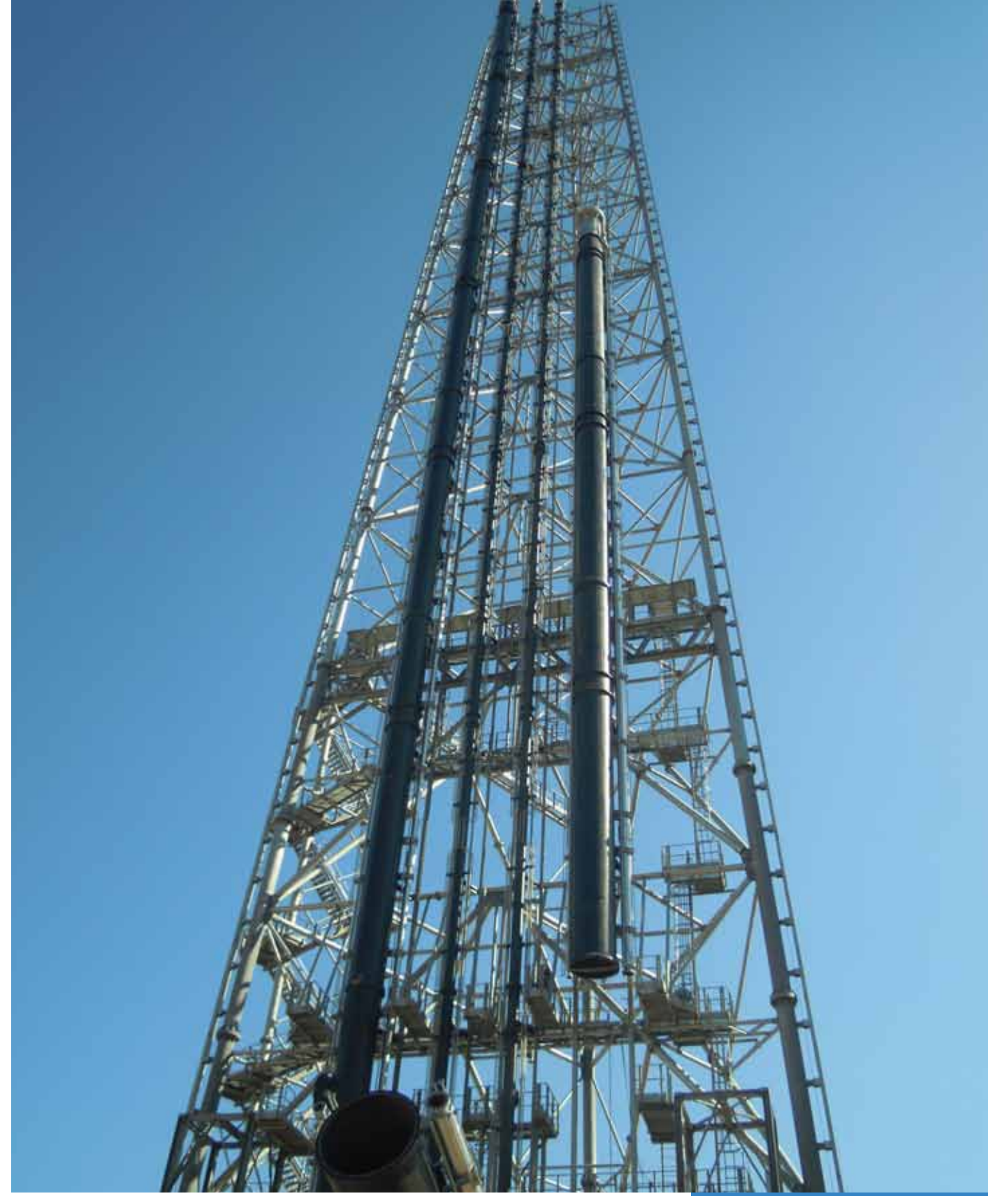
Demountable Derrick Structure during dismantling Cartagena, Spain
