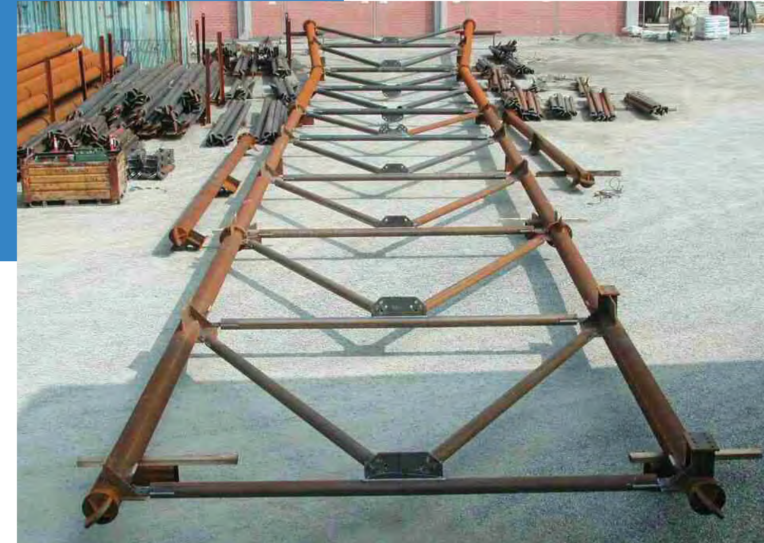
Trial Assembly of Derrick Structure
