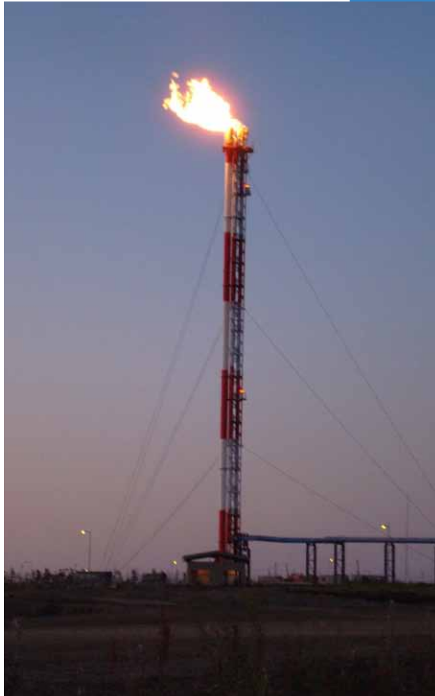
CSF HP & CAF LP Flare Tips on an 80m Guyed Derrick Sakhalin Island
