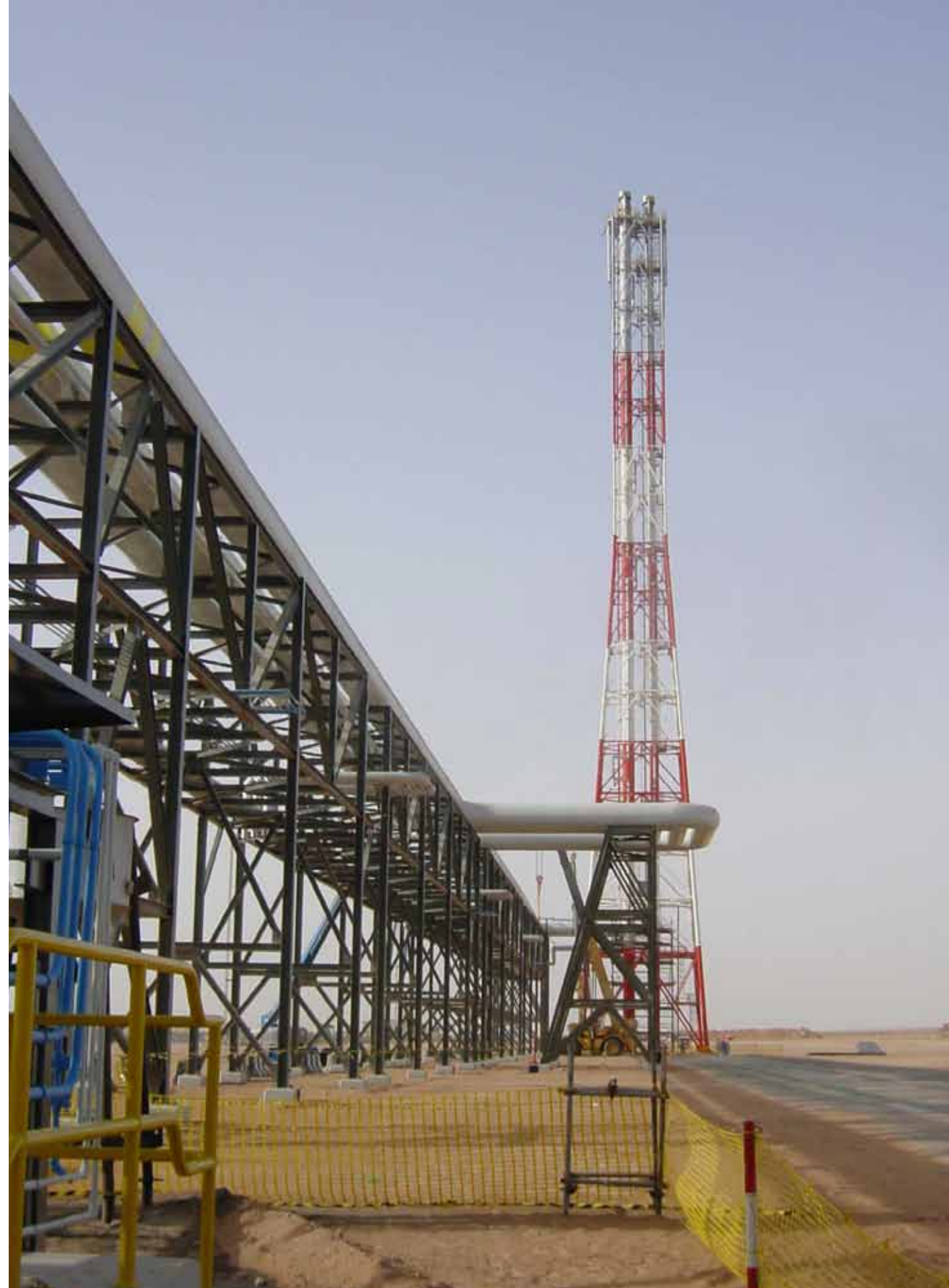
105m Fixed Derrick Supported Structure Ethylene project, UAE
