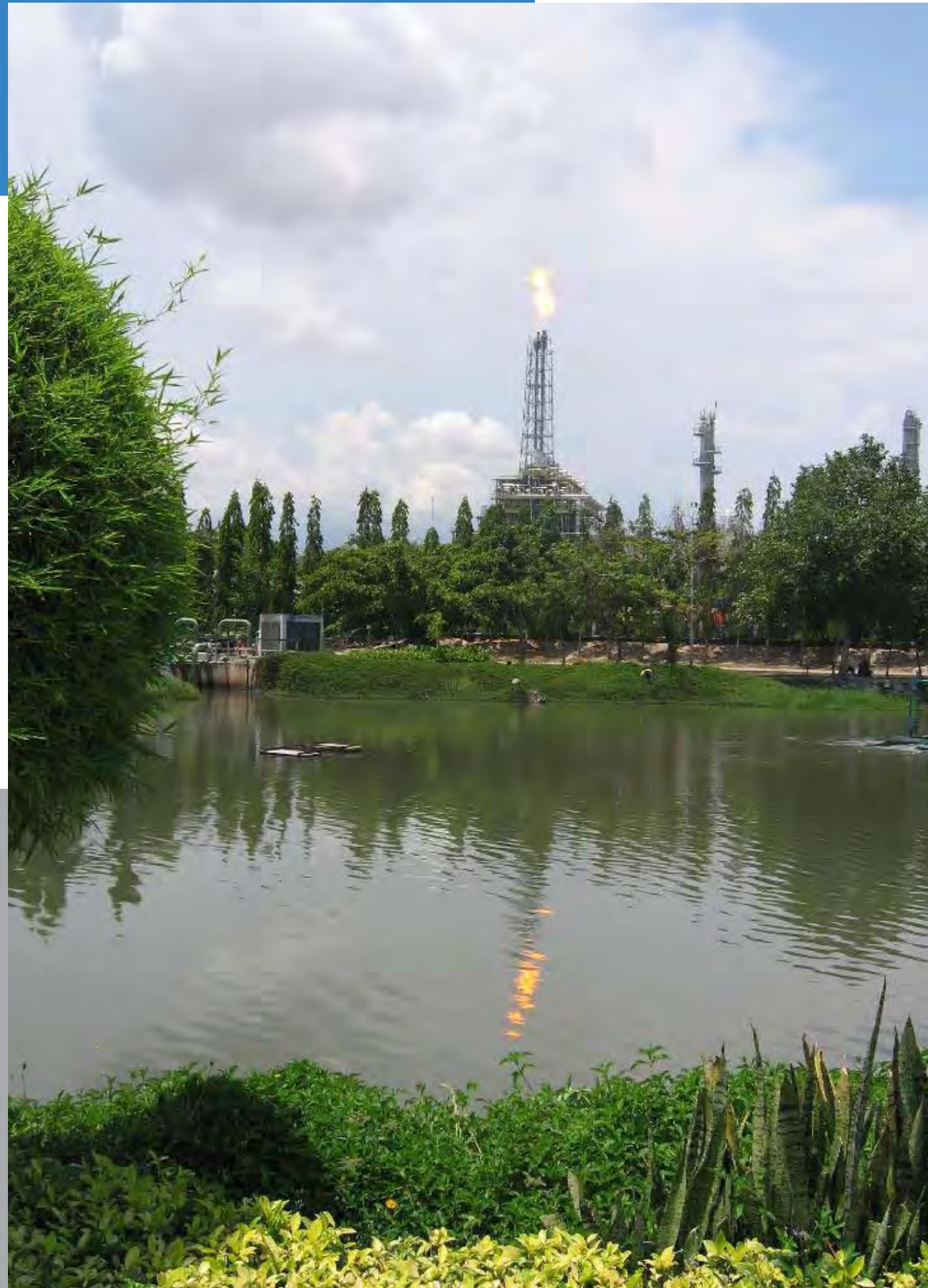
150m Demountable Riser Structure Supporting 3 smokeless flare tips in Thailand
